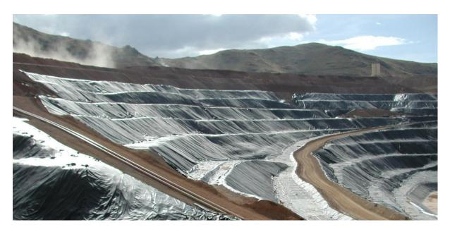
While HDPE liners have long been the default choice for mining applications due to their broad chemical resistance and low cost, PVC geomembranes offer compelling advantages that deserve serious consideration. This is particularly true for heap leach pads, acid lagoons, brine storages and other harsh environments where strong acids and UV exposure are prevalent.
