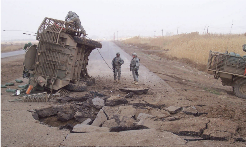
Figure 2. Damage to concrete road by an Improvised Explosive Device (IED)
