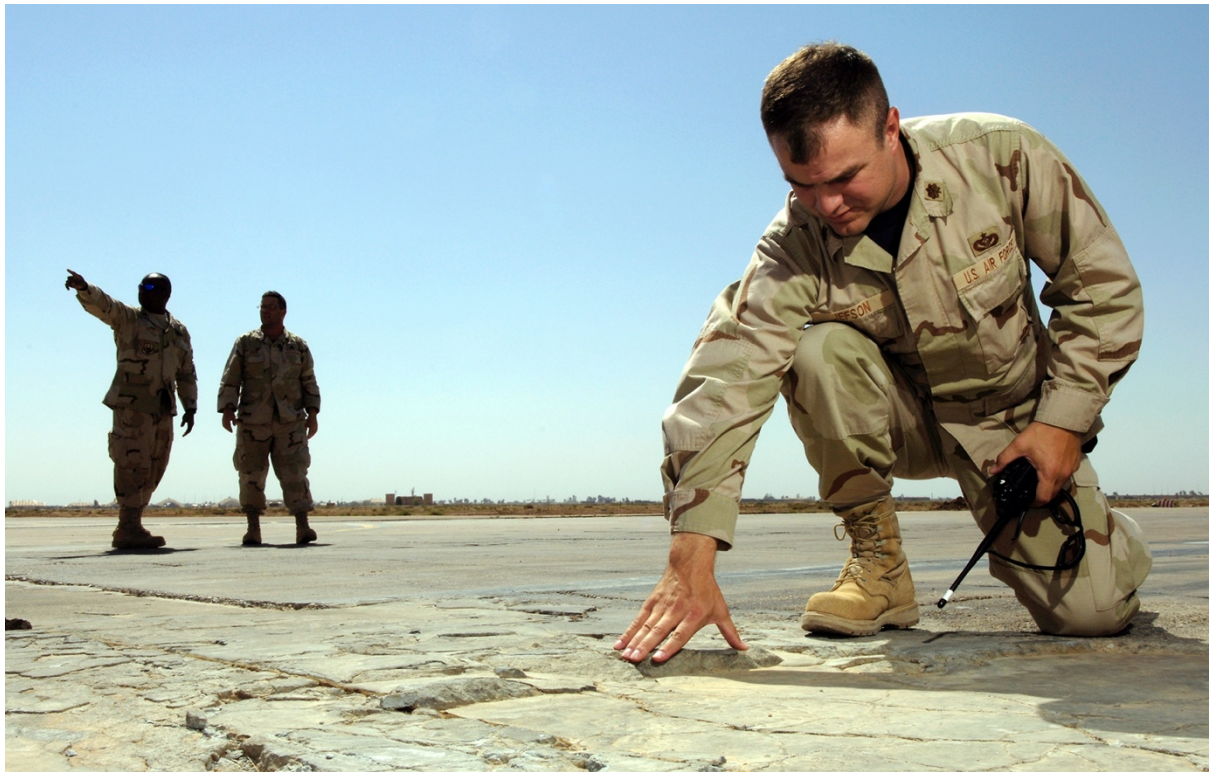
Figure 1. U.S. Air Force Engineer Inspecting Damaged Runway
