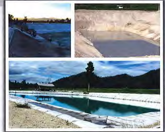
Application : Reservoir Reference Site : Concrete Agricultural Reservoir, Lampang, 5000 square meters
