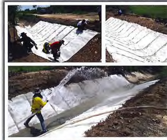
Application : Ditch Lining Reference Site : Agricultural Ditch Lining, Ratchaburi
