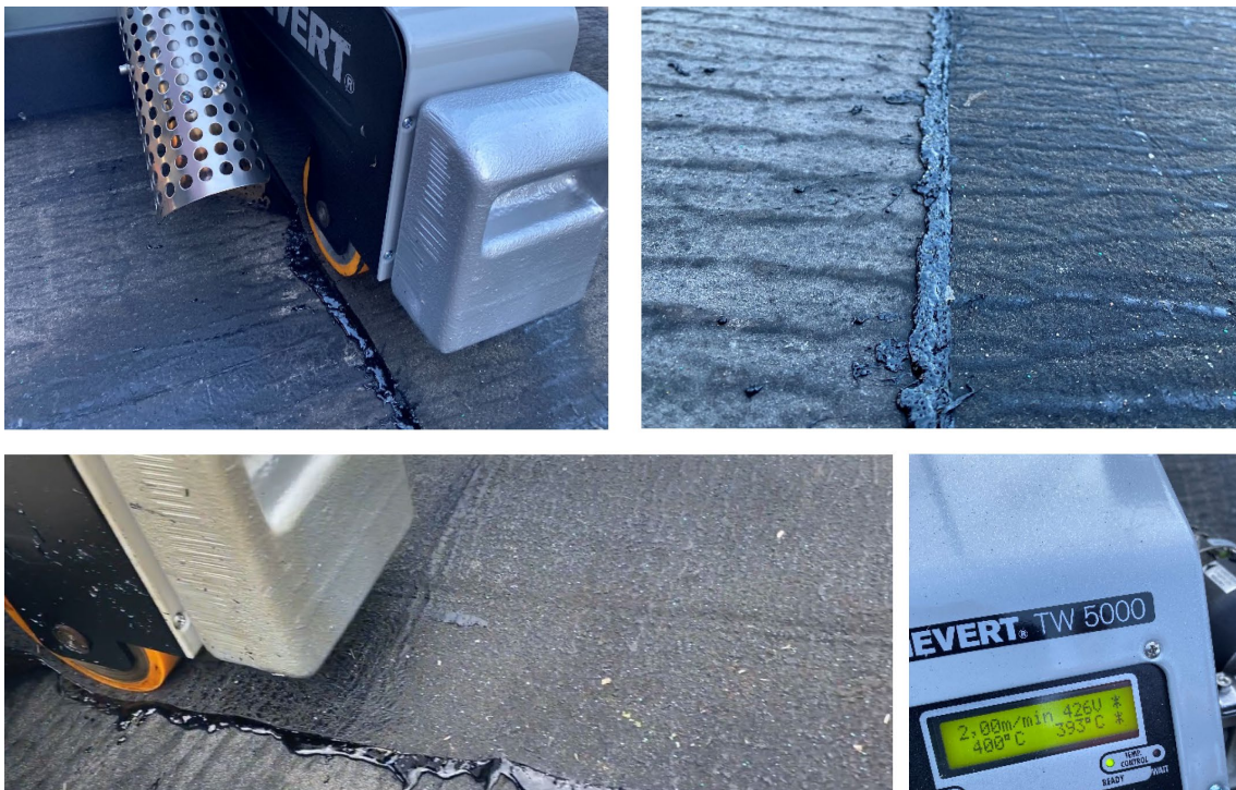
Figure 4: Axter's trials on a number of various electric welding machines showed that good seam strengths and complete sealing could be achieved.
