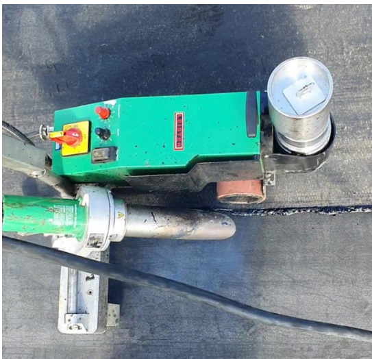
Figure 2. Note the good flow of bitumen from the welded seam which ensures excellent sealing and bonding.
