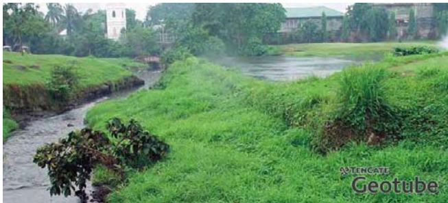
Picture 2: Golf Course Stormwater Protection (after)
