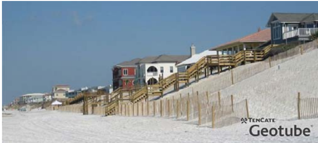
Picture 4: Hurricane Beach Repair New Jersey (After)
