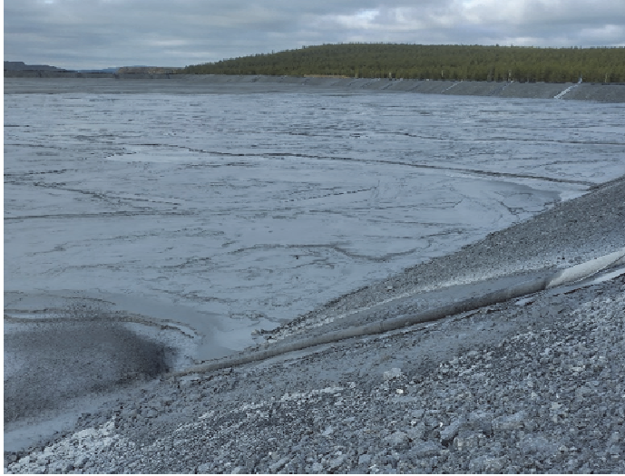
Fig. 2. A conventional method is hydraulically disposing of tailings as slurry into the wide tailings storage facilities using spigots or other pumping systems.
