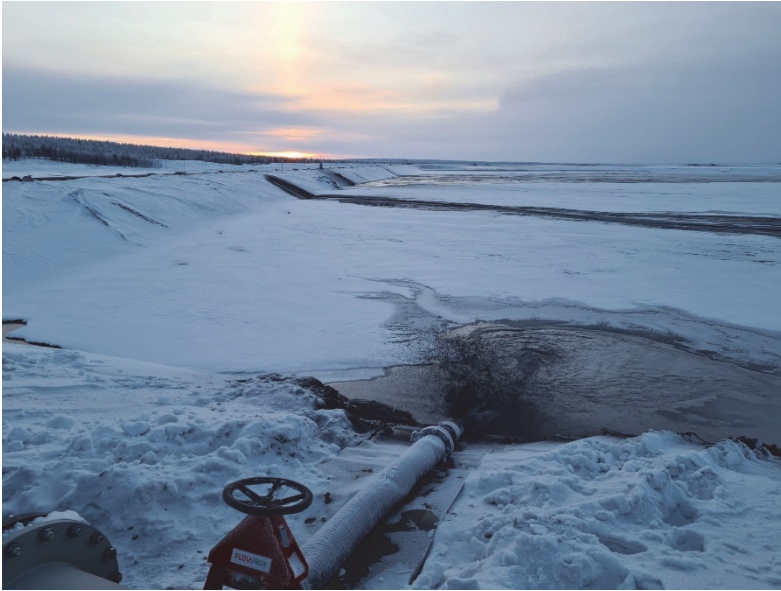
Fig. 4. The presence of snow and ice causes issues for the design and operation of tailings storage facilities (Photo: Johanna Holm Boliden Kevitsa).
