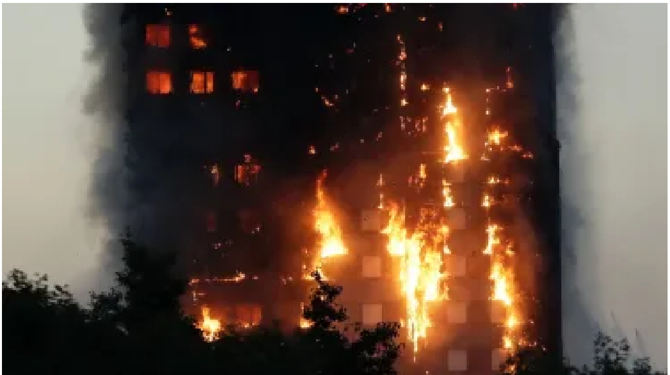
The Grenfell Tower fire in London in 2017 claimed the lives of 72 people.AP
