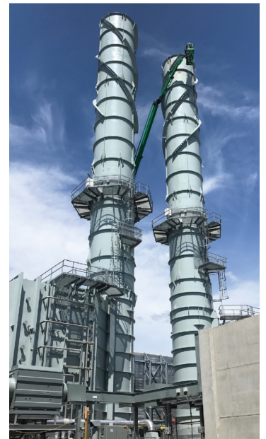
The coating on the finished stacks is designed to protect the steel at service temperatures of up to 500 F.
