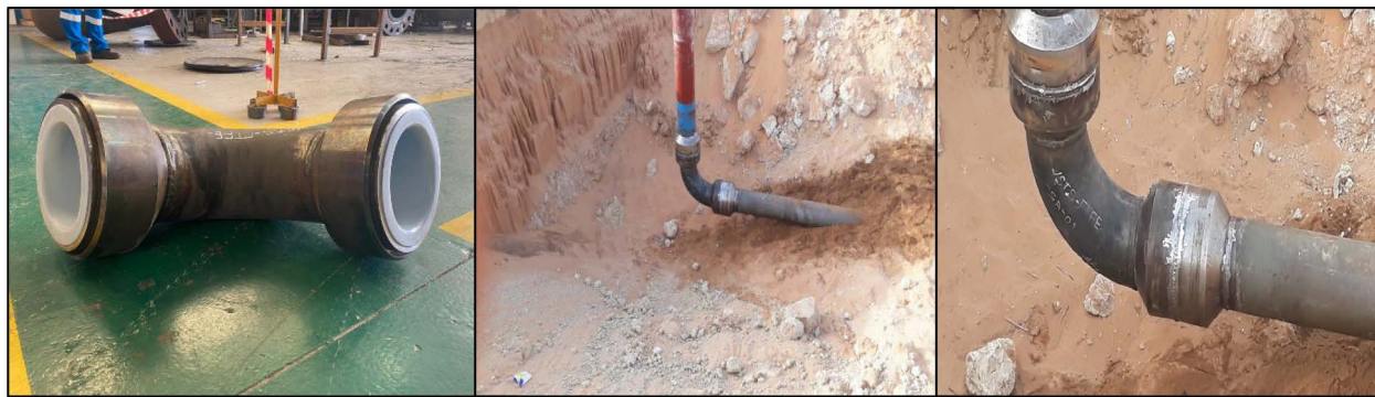
Figure 2—Ethylene Tetrafluora Ethylene roto-lined project at KHRS-151
