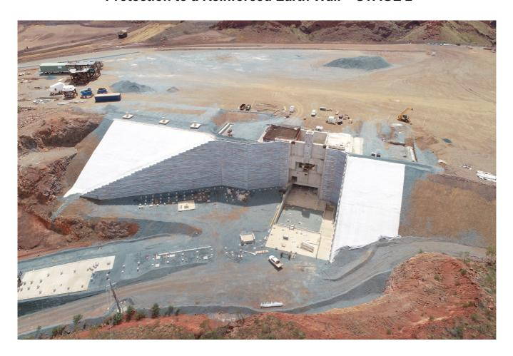
To continue on from a successful 1<sup>st</sup> Stage installation in December, 2022, Tiltex Australia's installation team have just completed Stage 2 of a major water infiltration barrier and ground surface erosion control to the ROM Wall Crusher project in Pilbara, Western Australia.
