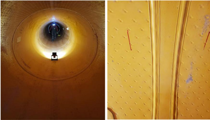
**Fig. 9** 1800 mm microtunnel with automatic welding of capstrip on right. Capstrip is unavoidable in precast pipe due to gaps too large to create a single bead
