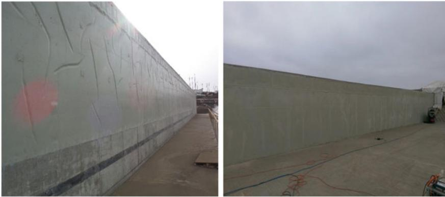
**Fig. 6** Anti-friction application that was not gapped and/or attached correctly. About \$250,000 repair on right
