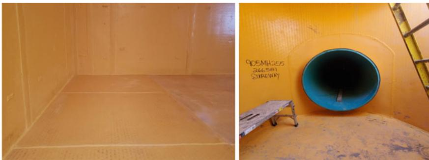
**Fig. 7** Vault (left) with wall gaps too large so more capstrip and welding than necessary. Manhole (right) with single pass weld joints and properly shaped penetration details
