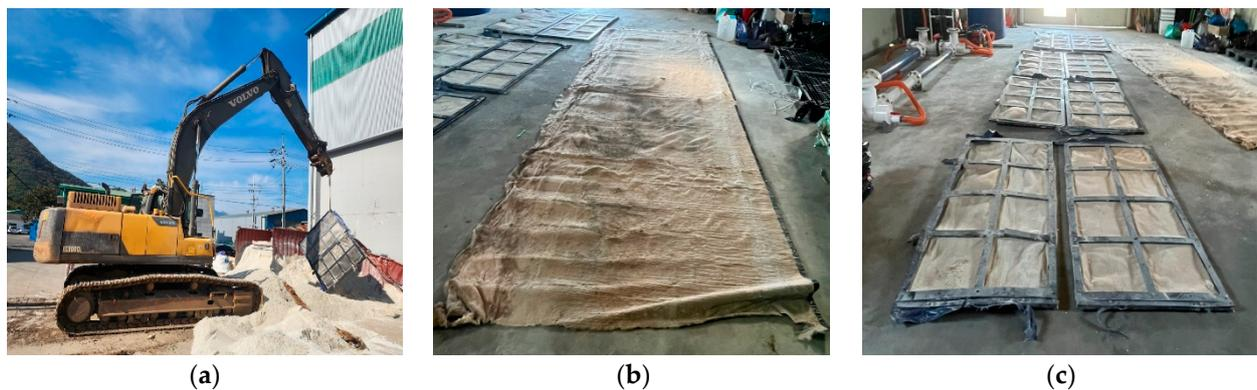
Figure 17. Inspecting the response of the smart liner: (a) demolition; (b) retrieved smart liner in the RSIM area; (c) retrieved smart liner in the PIM area.
