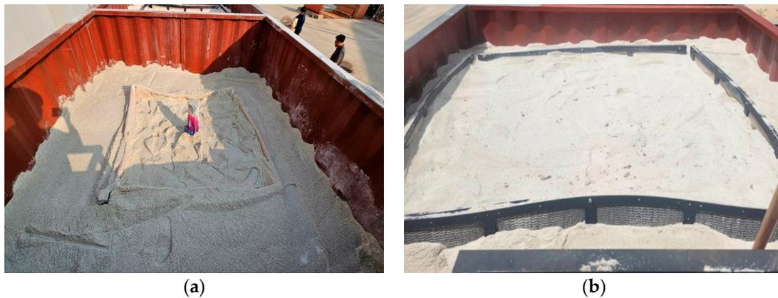
**Figure 8.** Backfilling using silica sand with construction method: (a) RSIM; (b) PIM.
