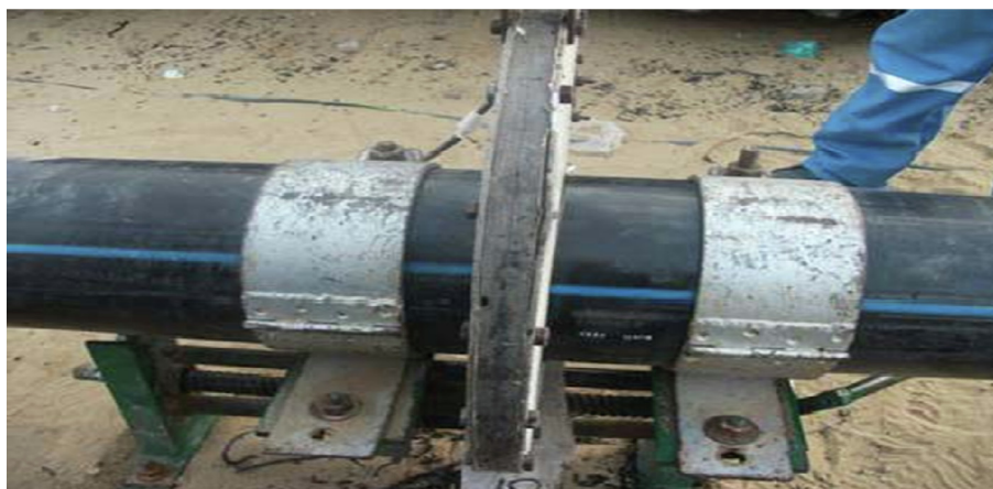
Fig. 4. Seaming of pipe with hot wedge welding machine.
