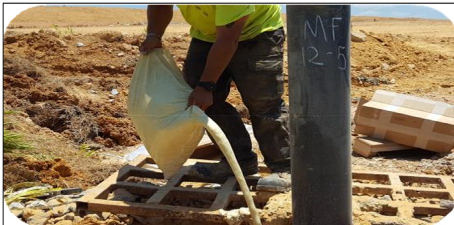
Fig. 5. hydrating bentonite to seal a well with pouring the casing.
