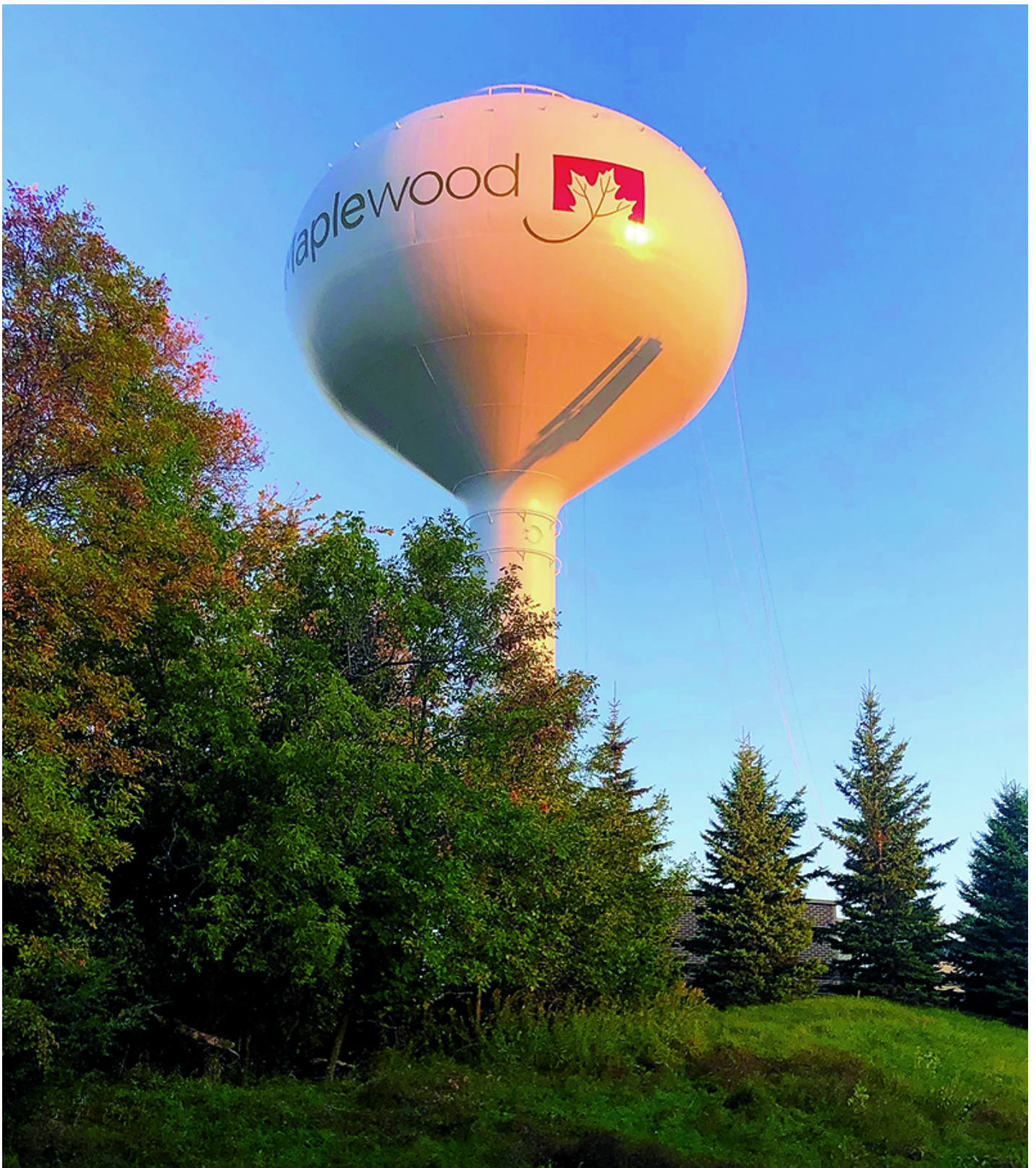
Figure 1: SPRWS selected a newly NSF/ANSI/CAN 600-approved, 100%-solids lining system for its 500,000-gallon Sterling Avenue water tower that helped the restored tank pass a discriminating water panel taste test on the first try. Courtesy of Sherwin-Williams Protective & Marine
