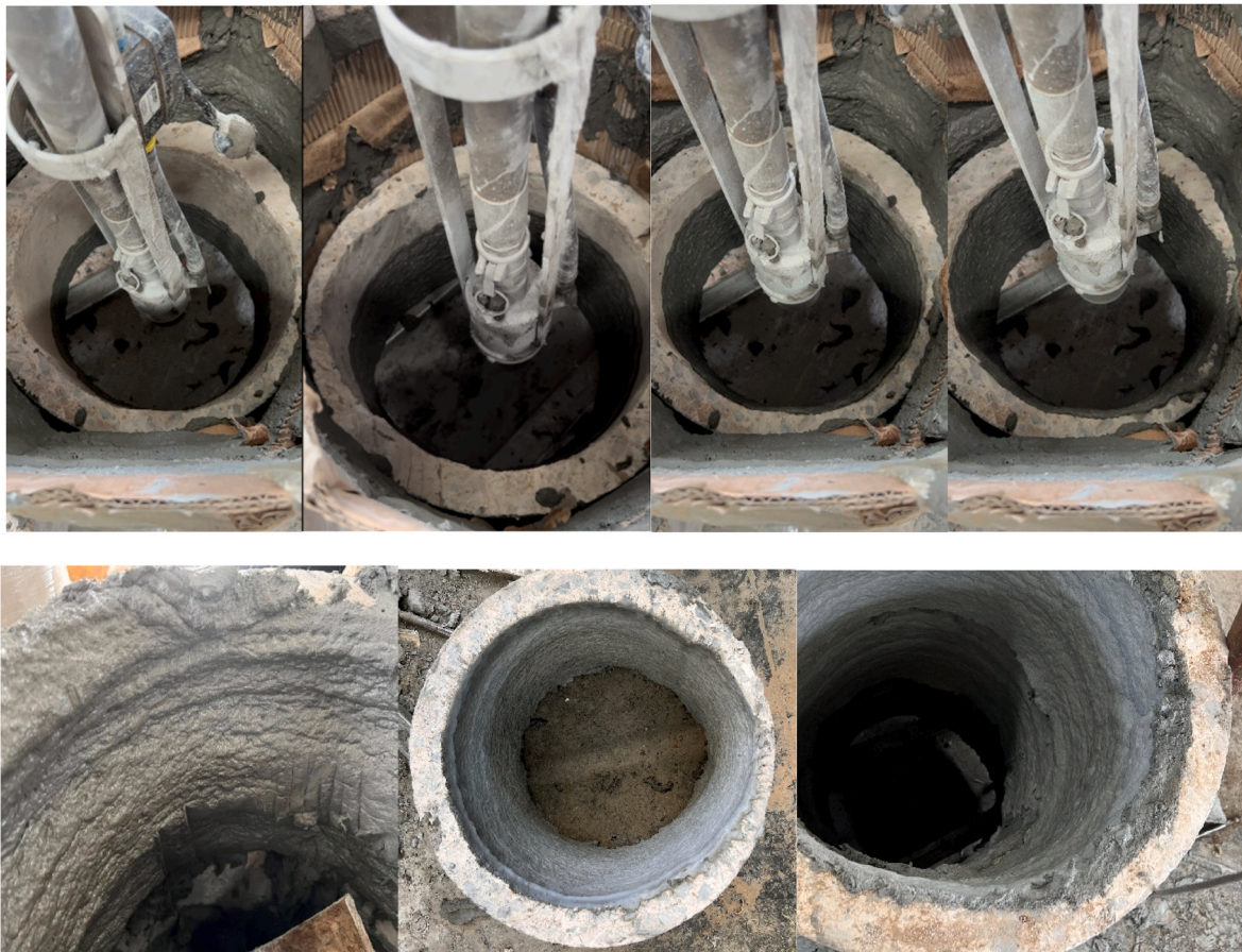
Fig. 16. Pipe spraying effect.
