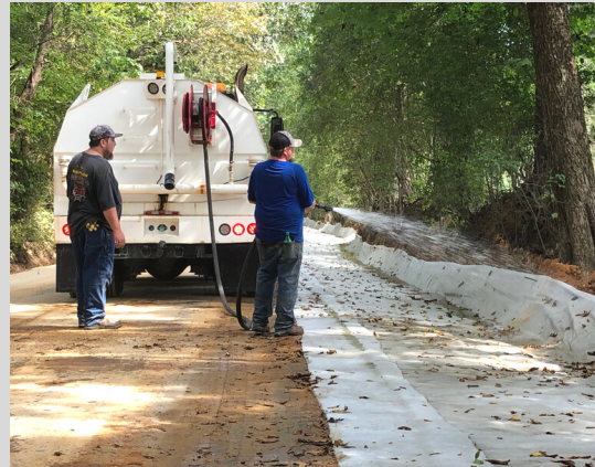
TRANSPORTATION Roadside Ditches
