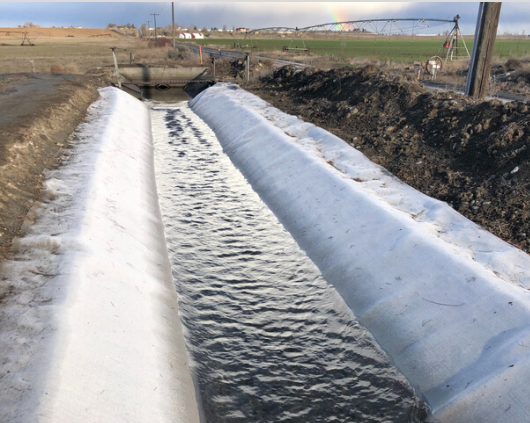
STORMWATER Canal & Culvert Repair
