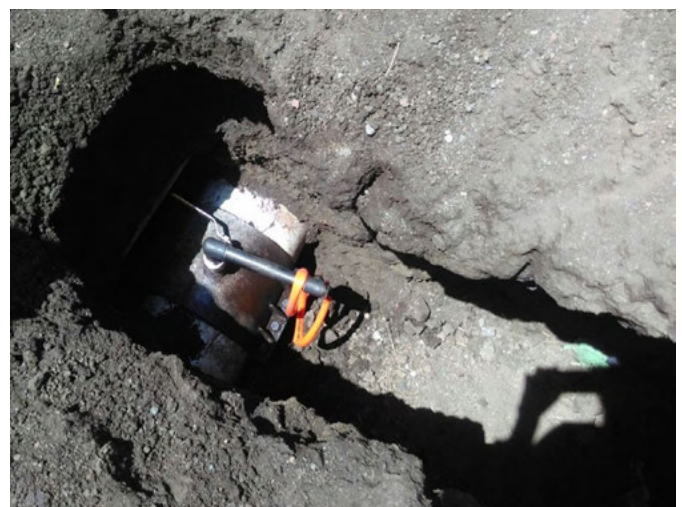
Figure 2: Hot-tap connected to a fuel pipeline in India.
