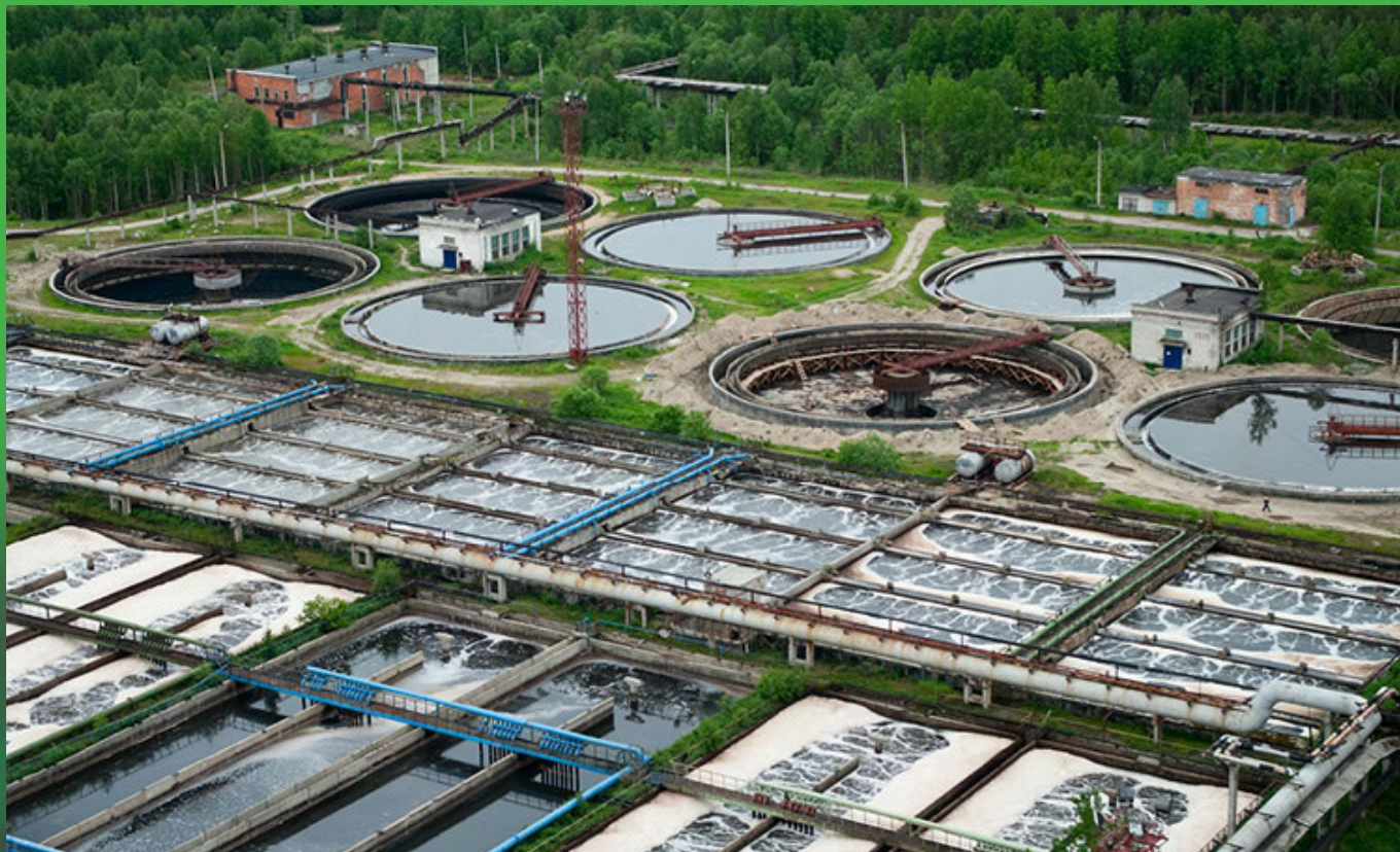
One of the topics of IDA: supply, disposal and treatment solutions for water and waste water (including training measures)
