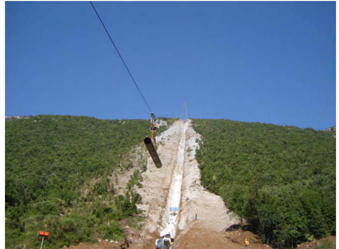
Figure 2: Transporting of the pipes to the intended location
