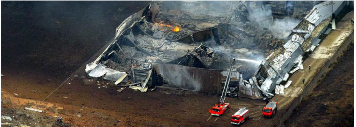
Figure 3: The Ghislenghien accident
