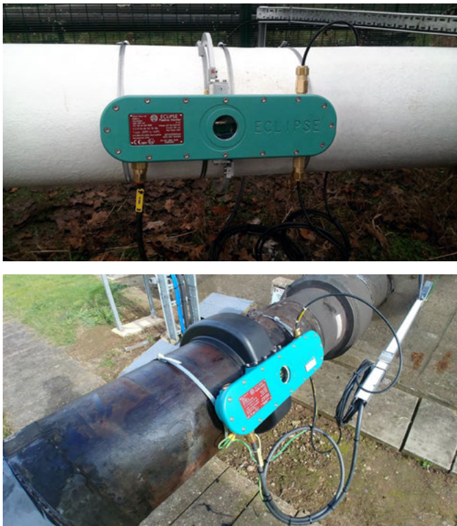
Figure 2: shows eclipse units installed on pipelines
