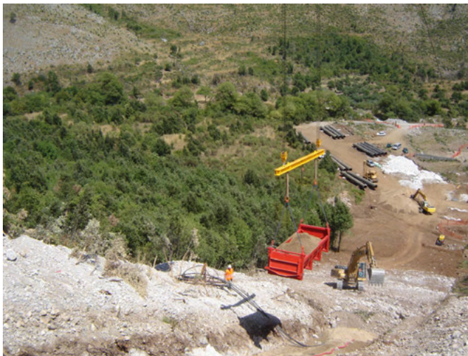
Figure 5: Transporting of a bulk for filling the trench
