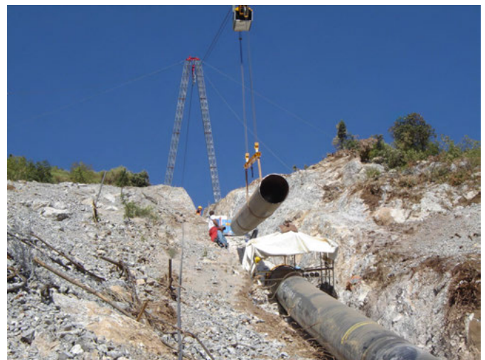
Figure 3: Fitting the pipes in the trench
