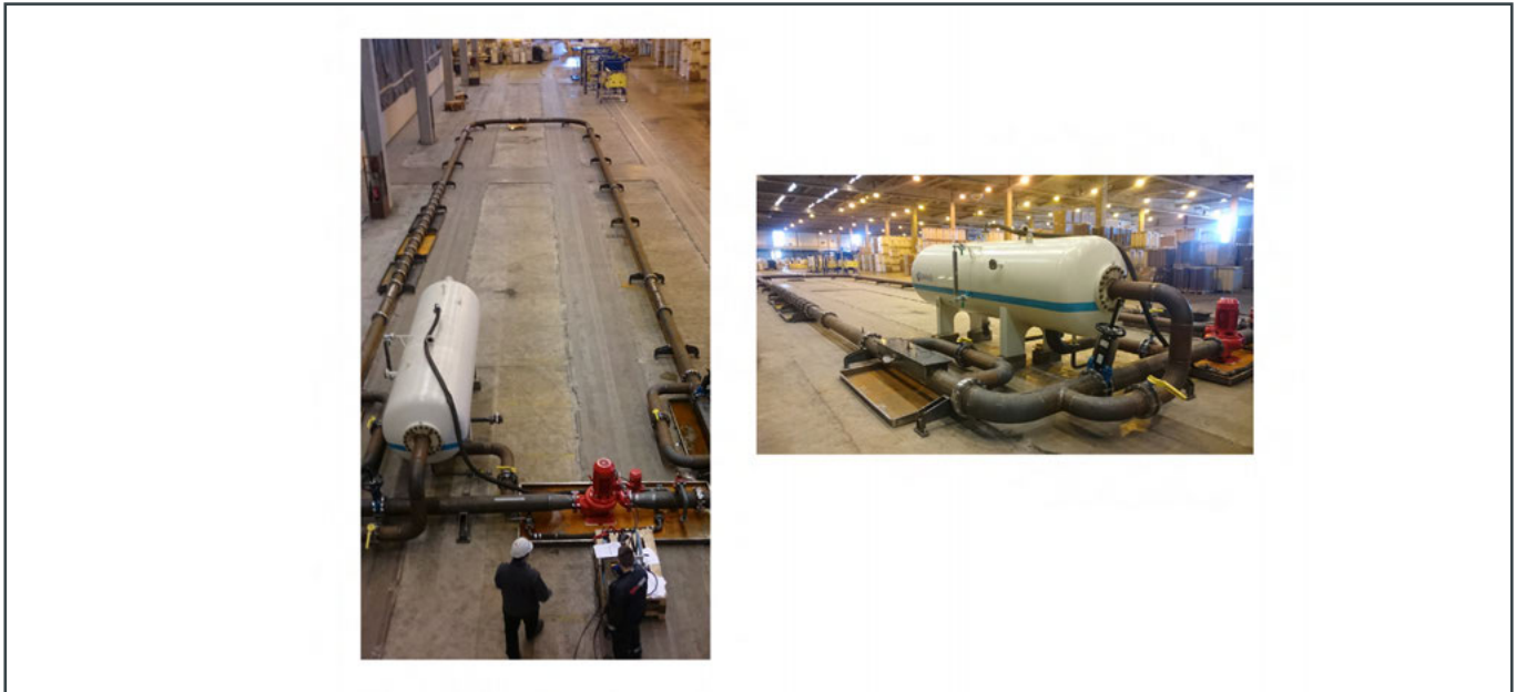
Figure 4: Flow loop test facility for 10" DILI tool.
