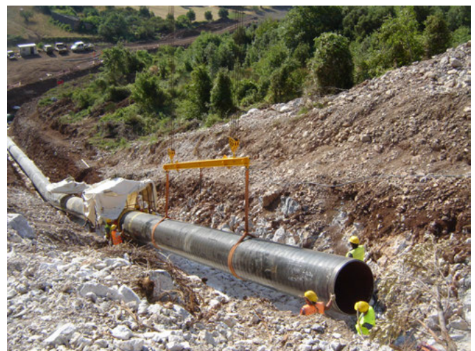
Figure 4: Fixing and preparation for the welding
