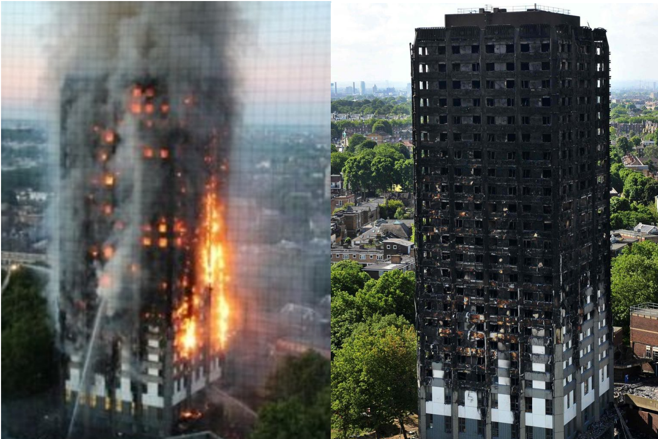
The notorious Grenfell Tower fire in London which spread via flammable cladding and left 72 people dead. The remains of the Grenfell Tower. Picture: AFP
