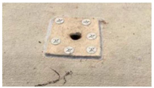
Photo shows a new puncture in a recently repaired GSC groyne
