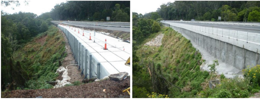
Fig. 6 Construction stages of the Geofoam construction for the acceleration lane
