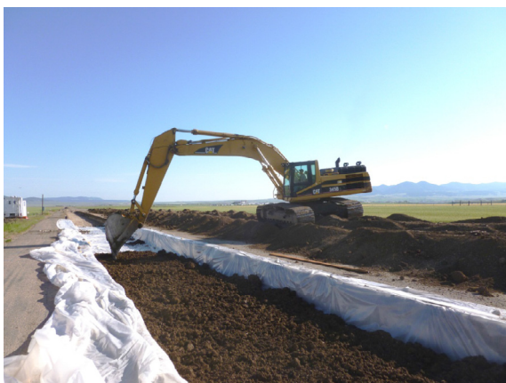
Fig. 4. Filling trench with prepared subgrade.
