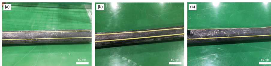
Fig. 1. Photos of buried pipelines in service; (a) 9 years in service, (b) 13 years in service, and (c) 18 years in service.
