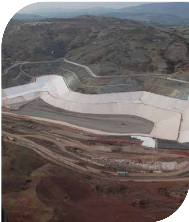
TURKEY MANISA GÖRDES STAGE 1 WASTE STORAGE FACILITY (META NICKEL) INTERDRAIN + TECHDRAIN 556.000 m 2
