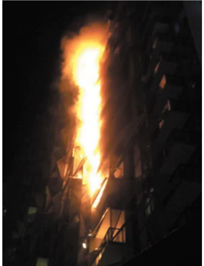
Flammable cladding alight on the Lacrosse building in Victoria’s Docklands.
