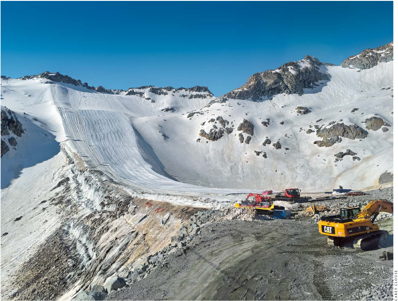
Figure 10 Crews assemble in preparation for summer blanketing at the Presena glacier in Italy, in the upper section of this ski run.
