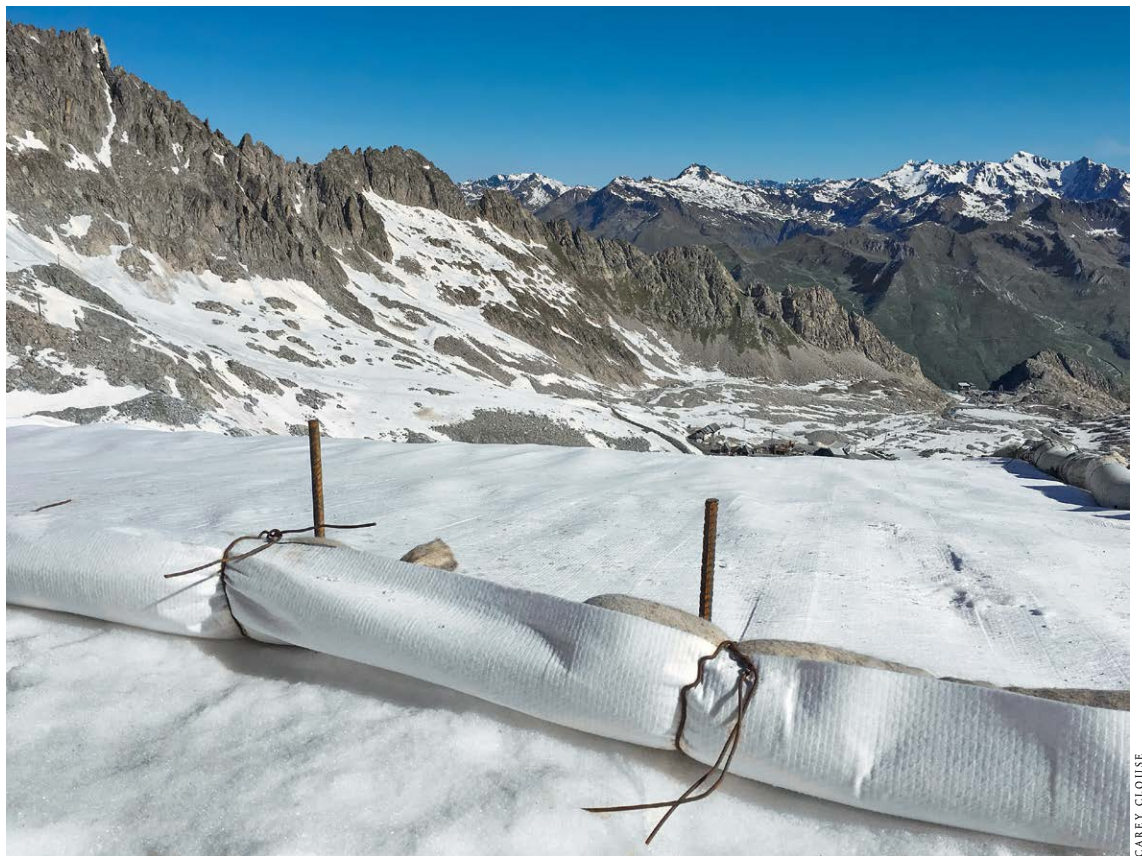
Figure 12 Rebar pins, sandbags and Polyfelt comprise the mountain attachment system at the top of ski runs.
