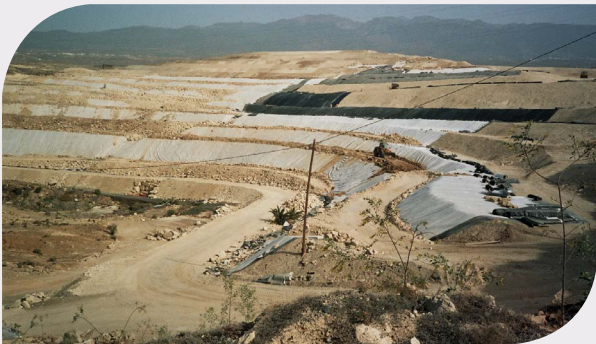
Indaver Landfill (Belgium) – 40.000 m 2 TECHDRAIN
