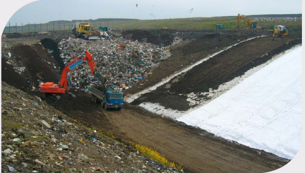
Ballealy Landfill (Ireland) – 200.000 m 2 TECHDRAIN
