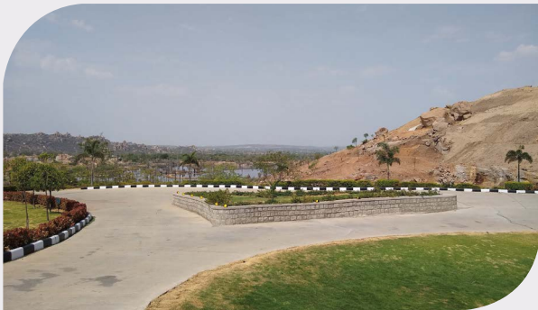
Hyderabad Landfill (India) – 550.000 m 2 CAPDRAIN
