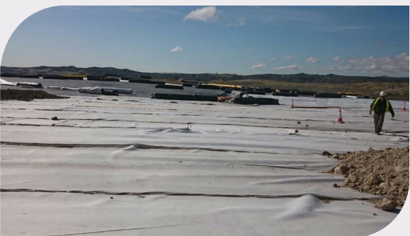
Valmadrid Landfill (Spain) – 433.000 m 2 CAPDRAIN
