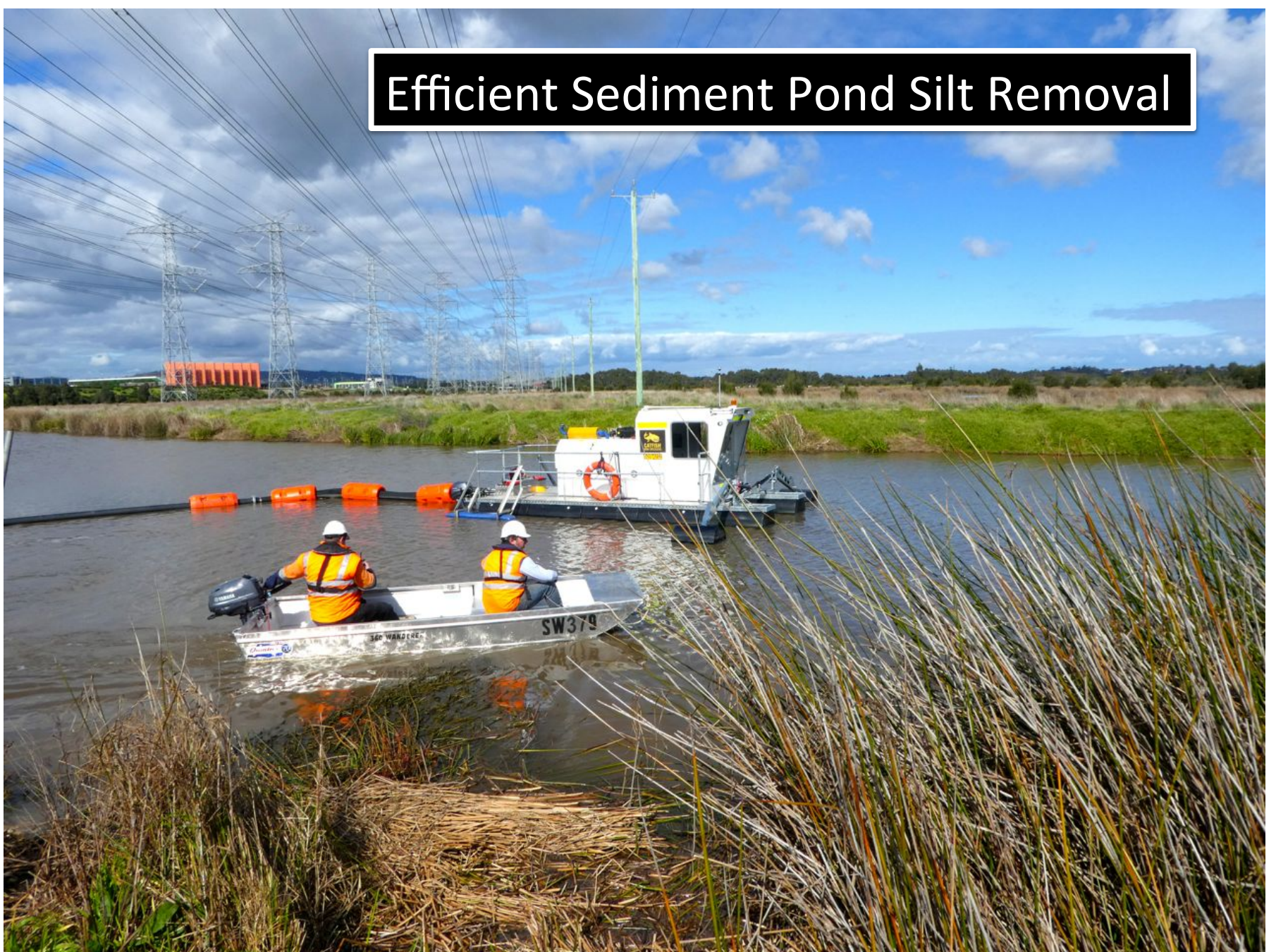
Mini-Dredgers Silt Removal & Dewatering
