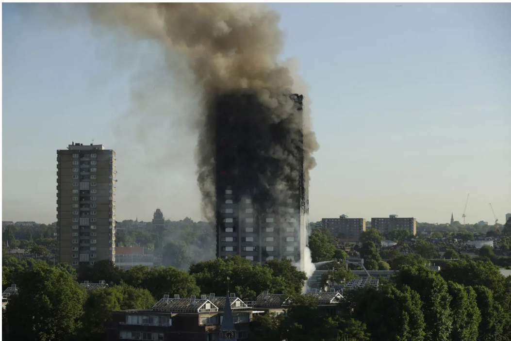
The same flammable cladding on Lacrosse was on London's Grenfell Tower (pictured). The public housing tower caught fire in 2017, killing 72 people. AP
