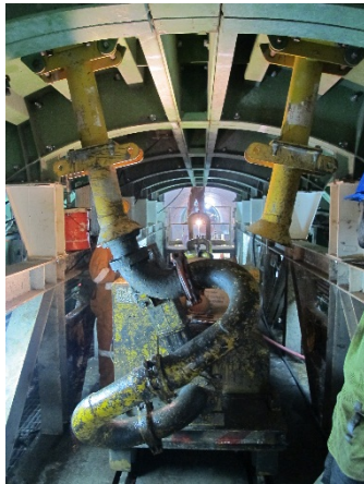
g – Pumping Concrete into Crown
