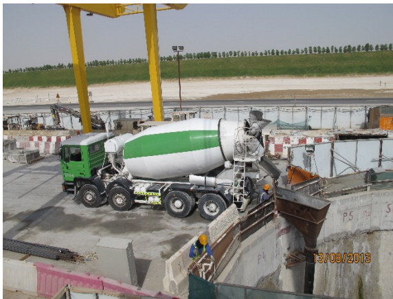
a – Concrete Discharged to Hopper
