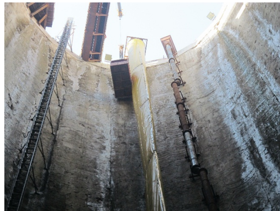
b – Hopper and Tremie Pipe in Shaft
