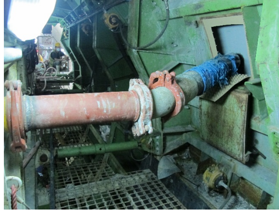
f – Pumping Concrete into Sidewall Port
