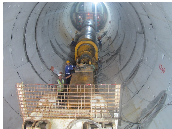
d – Transporting Concrete into Tunnel at Pour Location
