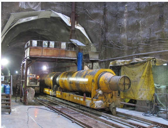
c – Discharging Concrete into Remixer Cars at Shaft Bottom
