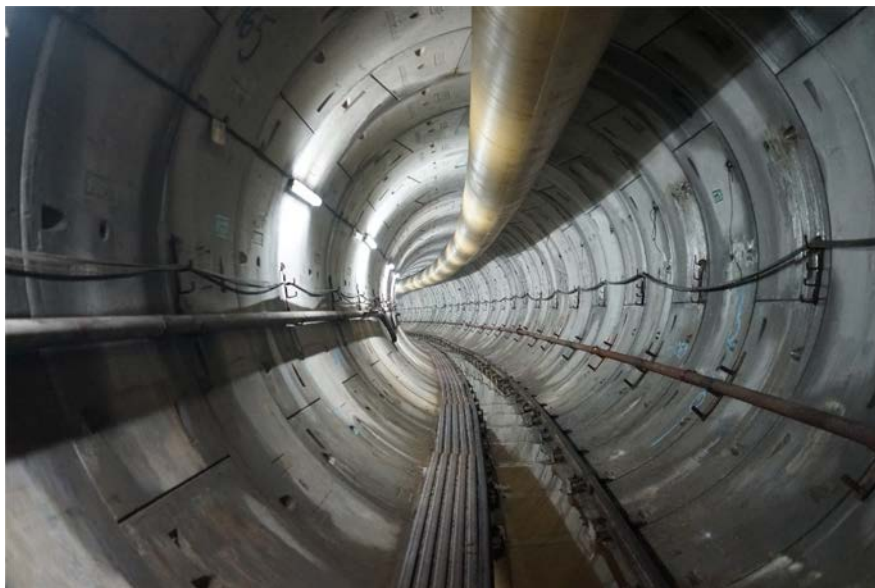
Figure 3. TBM Tunnel Segmental Lining (Contract T-01)
