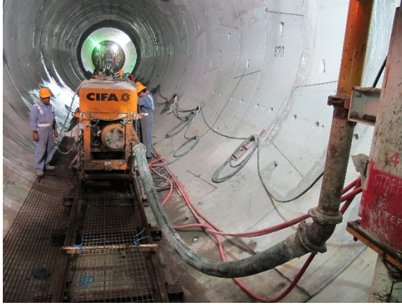
e – Pumping Concrete to Shutter
