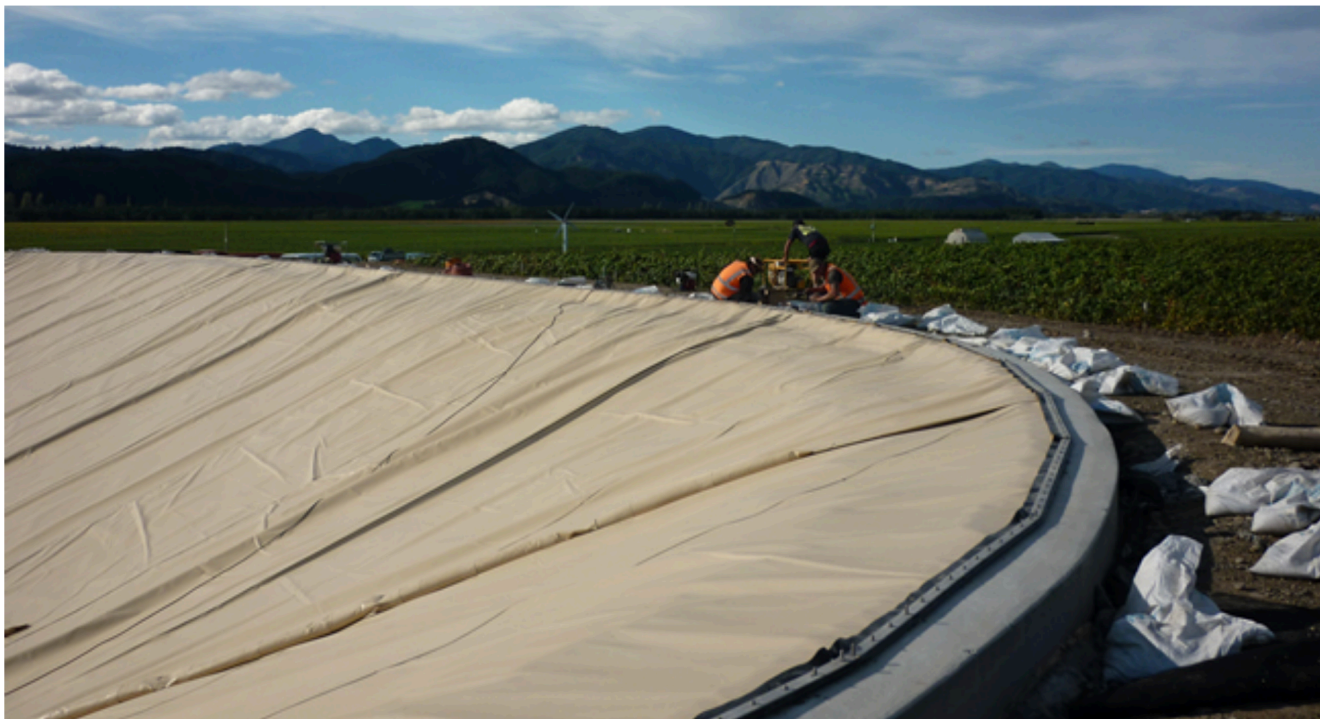
A "tension plate" floating cover system was used for the wastewater treatment pond. Here: a mechanical batten bar and rubber gasket system seals the polypropylene cover to the ring beam. Photo by Viking Containment .
