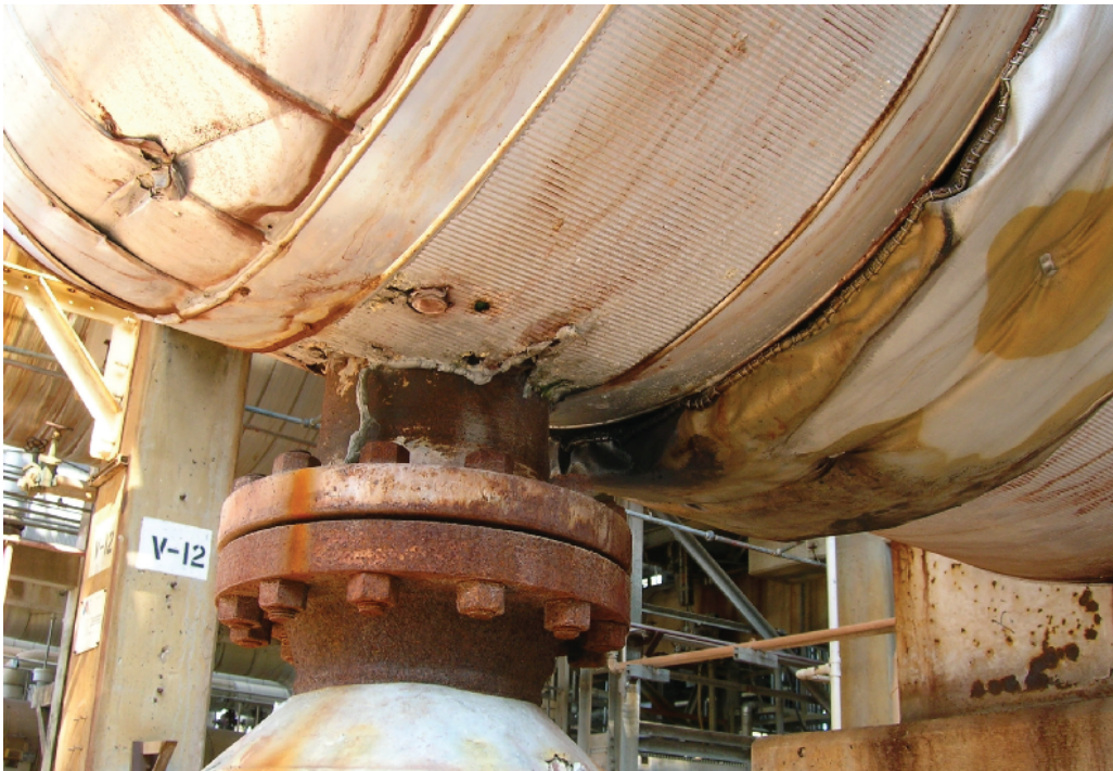
Fig. 4: Plant environment and acidic product leakage have eaten away the aluminum jacketing on this vessel—a clear indicator of moisture-saturated insulation.
