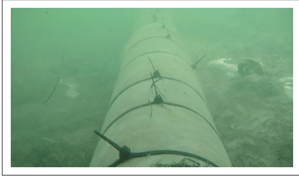
Figure 6. Underwater pipeline protection.
