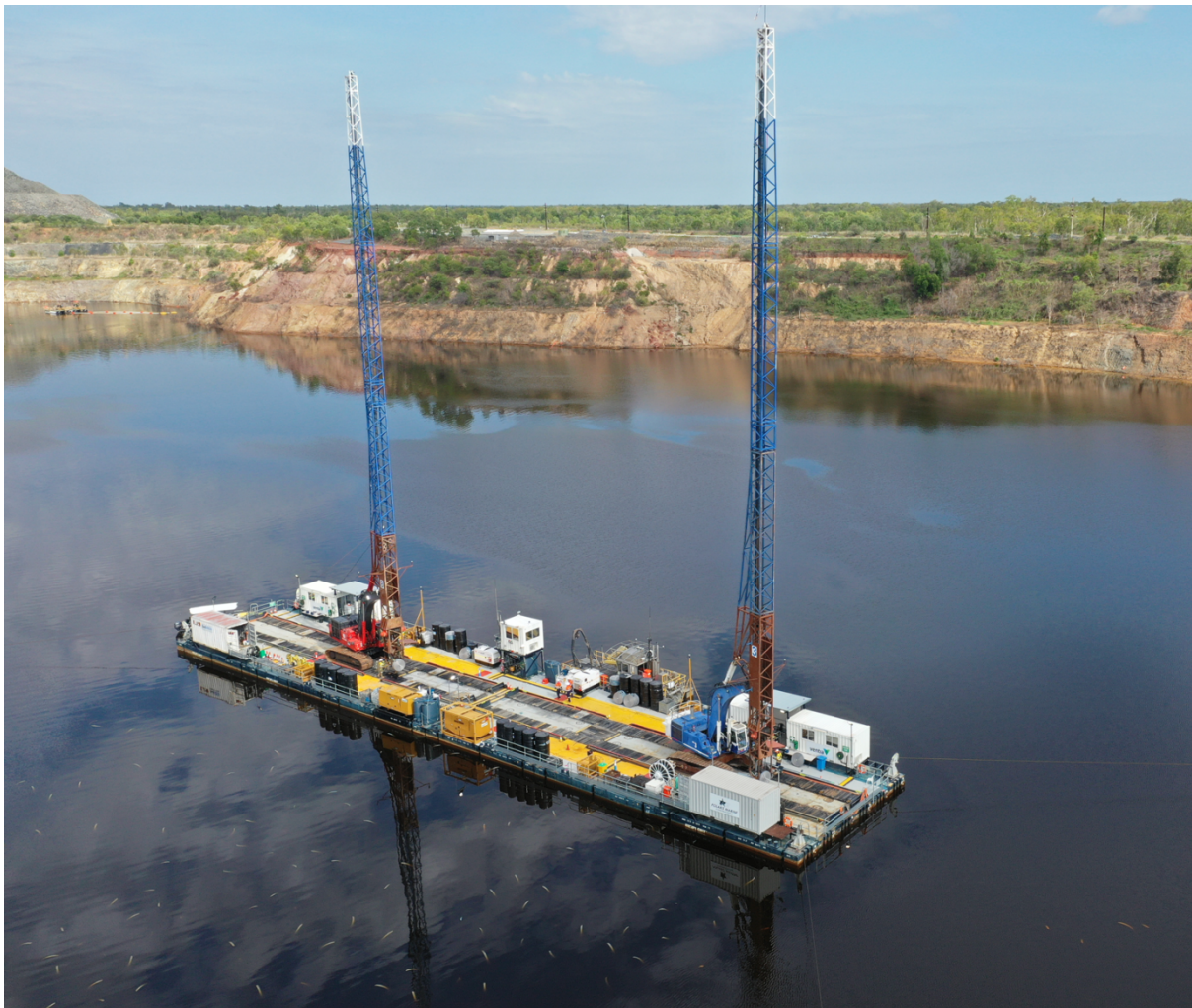
Figure 3. The PVD's were installed from a barge by Ventia https://www.ventia.com/
