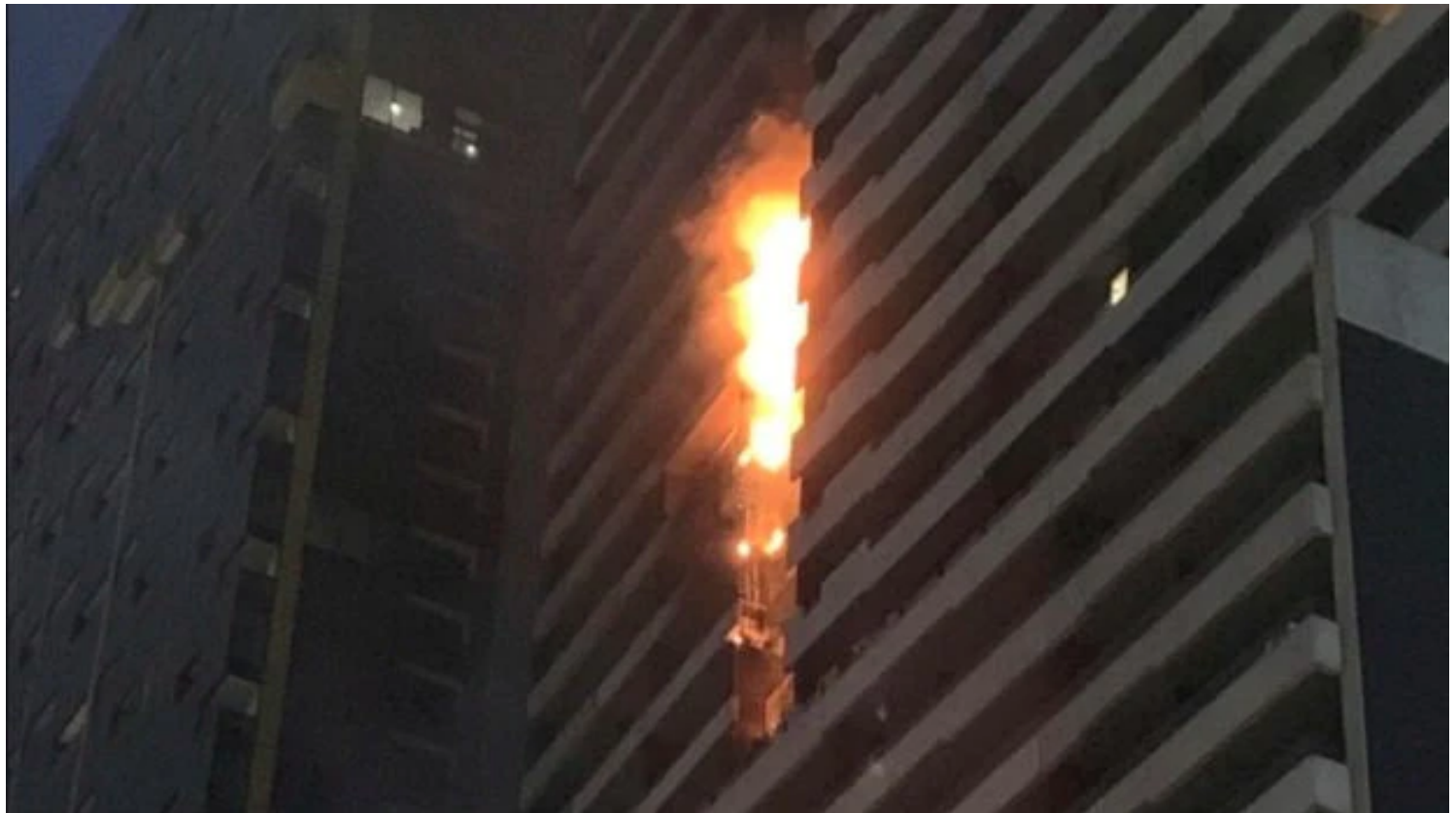
Flammable cladding, pictured at The Neo 200 apartment block in Spencer Street, has still not be removed from eight major Melbourne hospitals.
