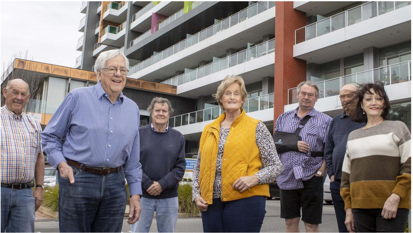
Residents of Air Apartments, in Eastwood, have concerns about flammable cladding on the Apartment building. Picture: NCA NewsWire / Kelly Barnes
