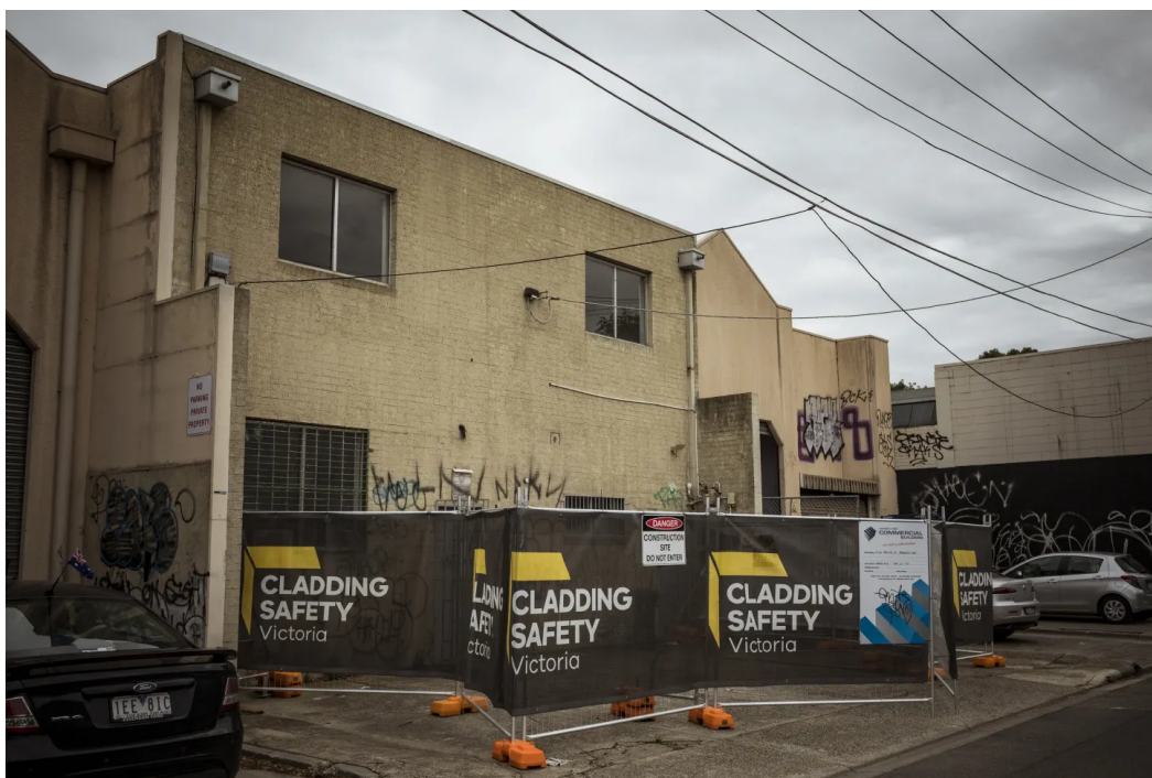
A building on Little Miller Street, Brunswick East. CHRIS HOPKINS
