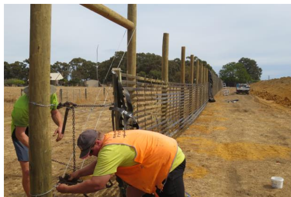
Tensioning the Parafence™ prior to connecting to the posts
