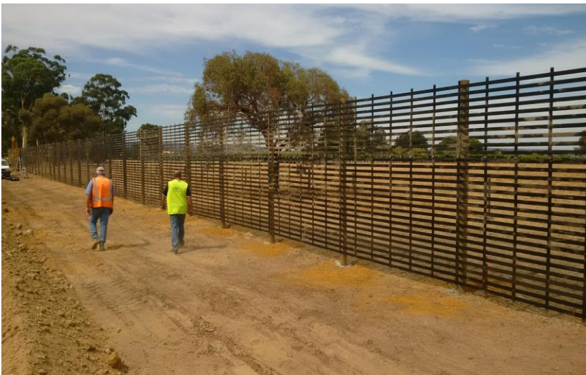
The completed 900m long x 2.8m high Parafence Windbreak Fence
