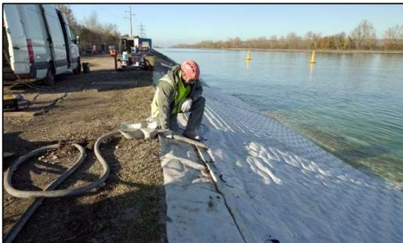
**Figure 13.** Grouting the mattress
