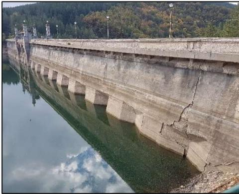
**Figure 1.** Deteriorated upstream face at Studena dam
