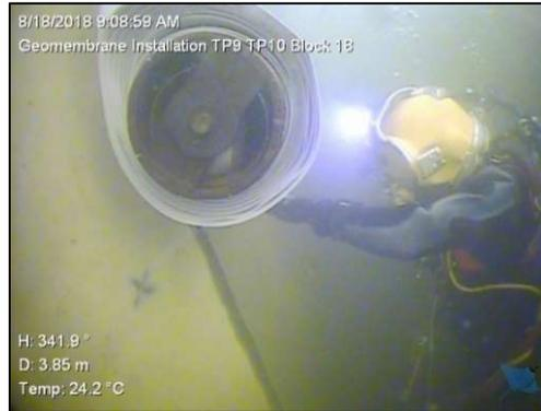
**Figure 5.** Unrolling of a geomembrane sheet underwater, over the 2000 g/m<sup>2</sup> non-woven geotextile
