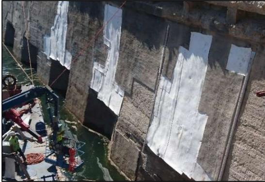
**Figure 4.** The 2000 g/m<sup>2</sup> non-woven geotextile is installed on the concrete after removal of the unbonded shotcrete, in the dry and underwater
