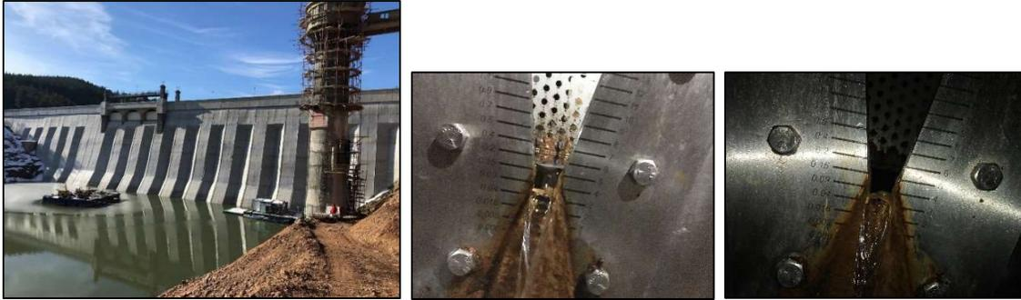
**Figure 8.** The works during a low water level period, and total leakage from the two drains
