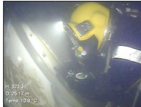
**Figure 7.** Diver connecting the two tensioning profiles underwater
