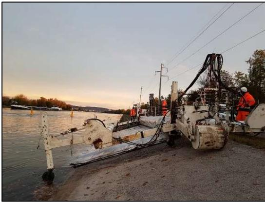
**Figure 11.** The empty mattress deployed to underwater placement
