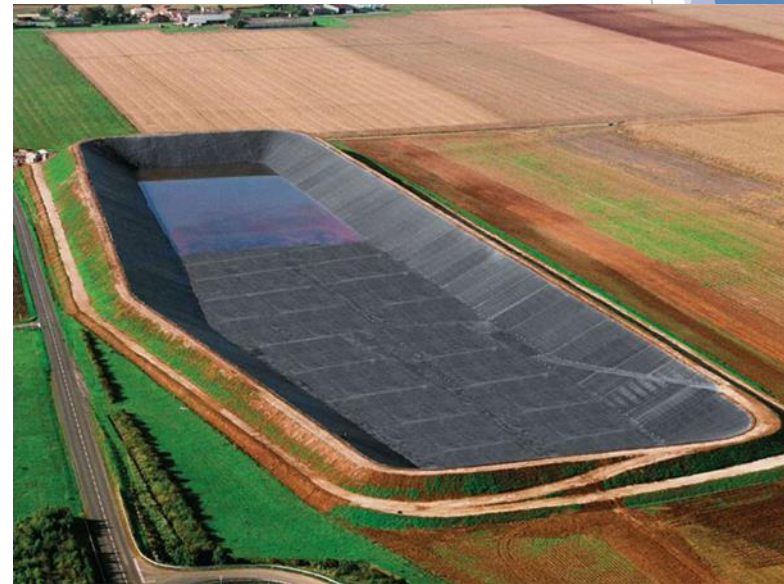
<Landfill preparation installed geomembrane liner>
