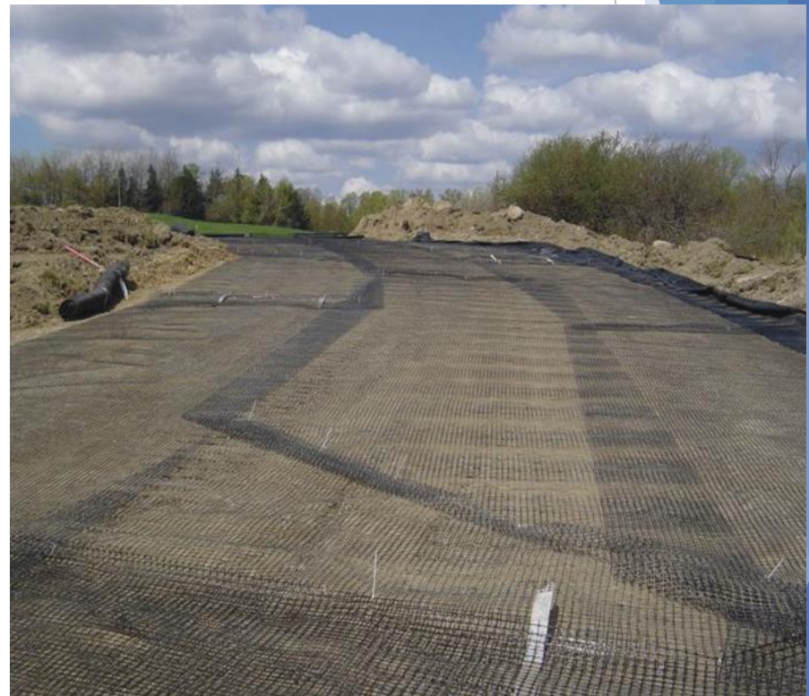
Representative geogrid and installation
