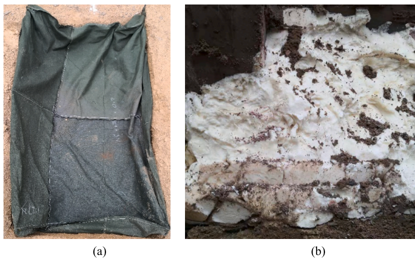
Fig. 6. (a) Preset of grouting bag (b) Effect of polymer grouting rehabilitation.
