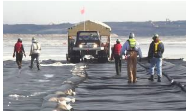
Figure 4. Placement of geotextile on frozen tailings pond.
