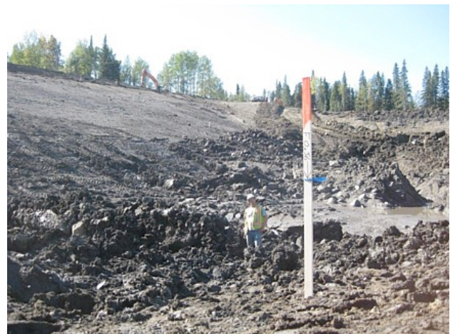
Figure 5. Subgrade preparation in wet conditions.
