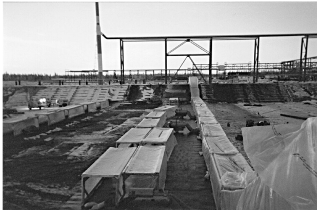
Figure 3. HDPE installation using temporary shelters.
