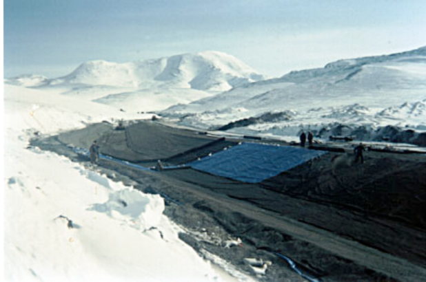
Figure 1. Winter install of RPE stream diversion in Alaska
