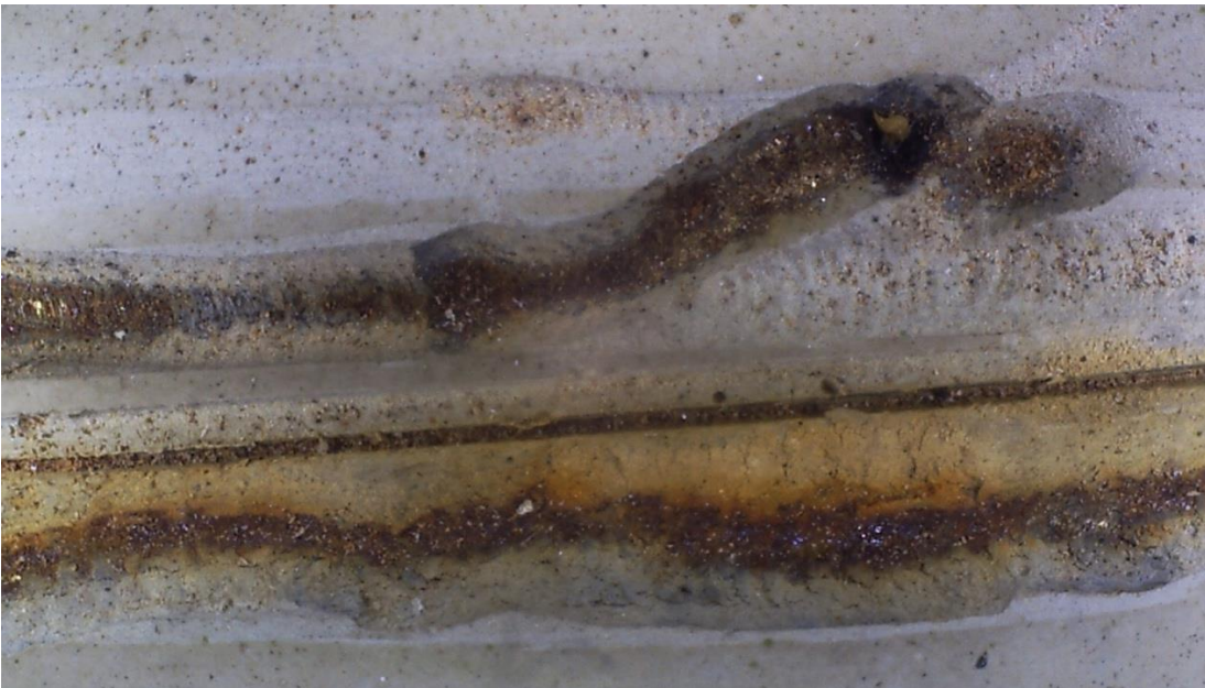
Above - Corrosion shown under 3.5x magnification
