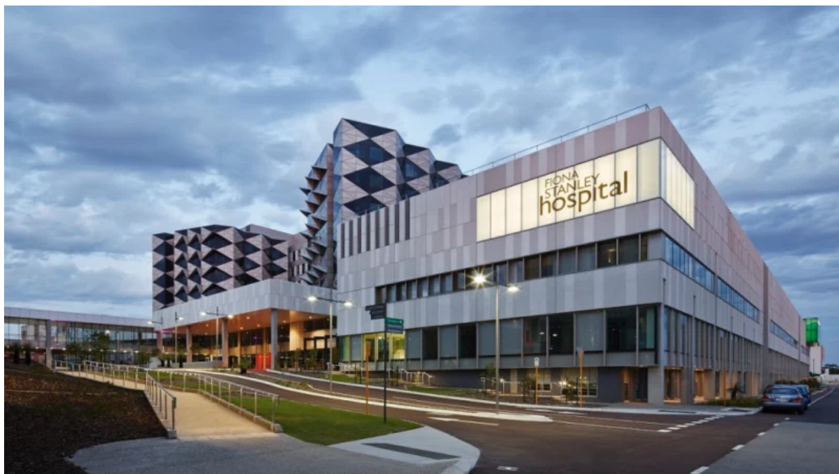
Fiona Stanley hospital was built with potentially dangerous cladding. PETER BENNETTS / FIONA STANLEY HOSPITAL DESIGN COLLABORATION
