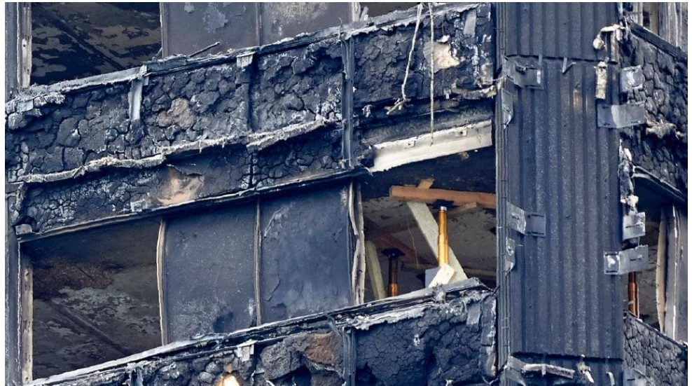
The charred remains of cladding are pictured on the outer walls of the burnt out shell of the Grenfell Tower block in north Kensington, west London. Picture: Niklas Halle'n
