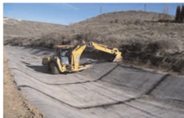
Figure 5. Traffic of heavy equipment for maintenance Yakima (Washington State USA).
