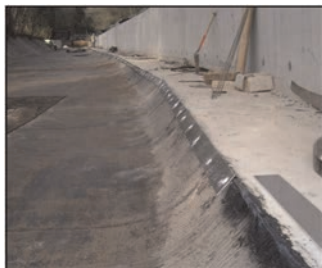
Figure 4. Canal in UK along deep slope.
