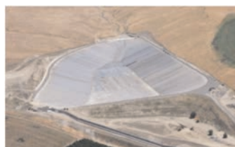
Figure 7. Wasteway No.5 Regulation Reservoir, feeding Yakima and Roza Districts Irrigation canals.
