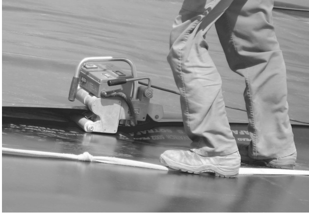
Figure 17.1 Photograph of seaming of HDPE geomembrane liners using a wedge welder (side view). Reproduced by permission of Sotrafa
