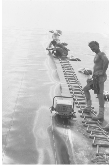
Figure 17.14 Photograph of a wedge welder seaming HDPE geomembranes on a steep slope. Reproduced by permission of NAUE
