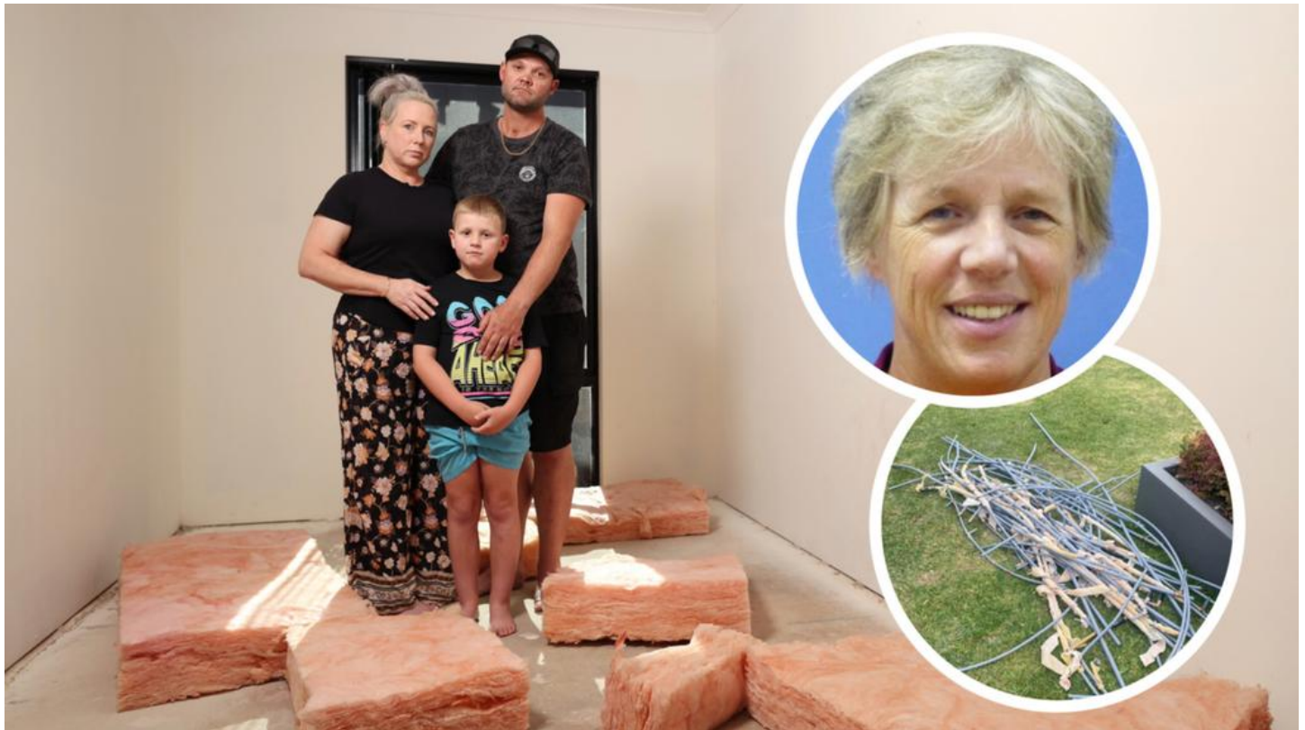
📷 Main image: Chris and Sarah Lyne with their son Nate (7) in one of the damaged rooms of their house. Top right: Outgoing WA Building Commissioner Kristin Berge. Bottom right: Some of the defective pipes stripped out of homes. Credit: The West Australian
