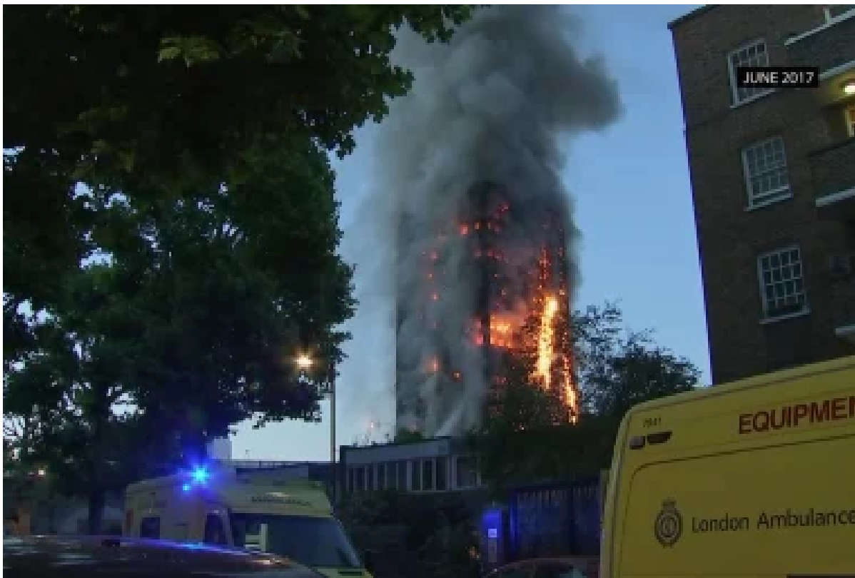
The devastating fire at London's Grenfell Tower in 2017. AP
