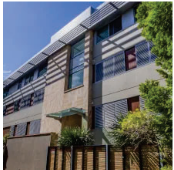
Owners of the 17-unit Shore Apartments in Sydney's Dolls Point are leading the action the against the Alucobond
