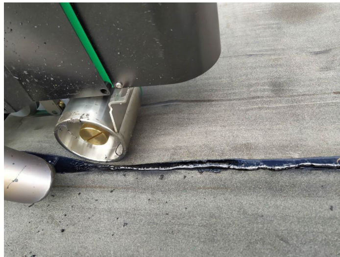
Flameless welding of Coletanche BGM for landfill capping. Queensland
