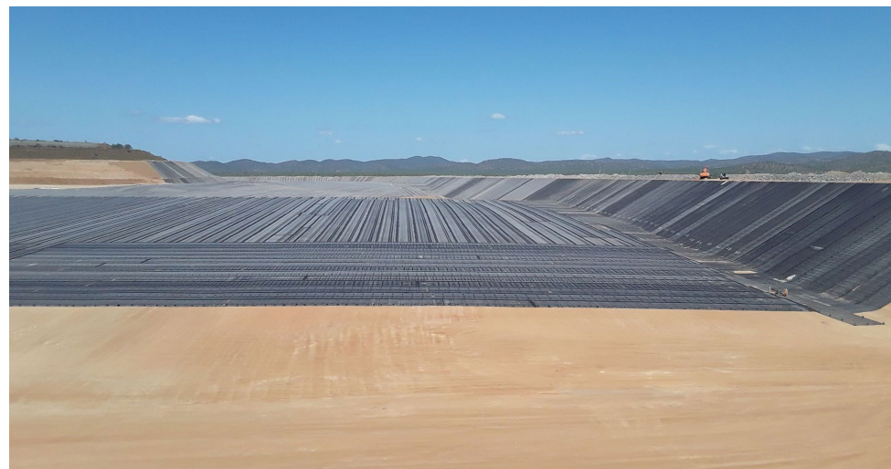
Gold tailings storage facility QLD
